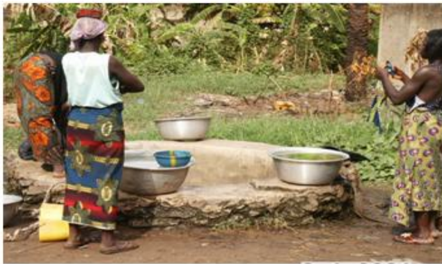
Photo 1: Well installed in a Unsanitary environment in Bêtou Shooting: LANDEOU, December 2018
