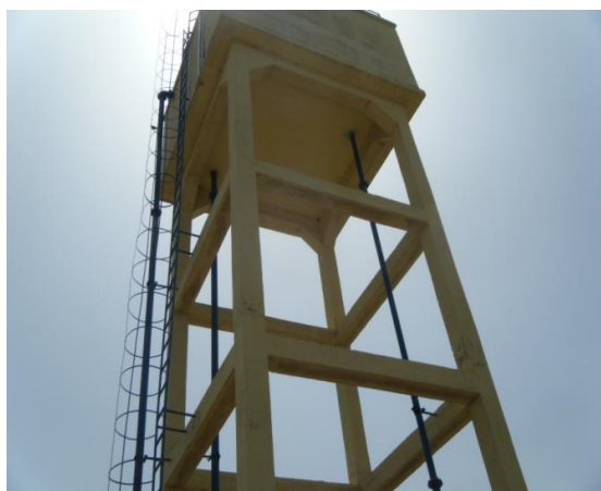
Photo 4: Water tower in the district of Goumori
