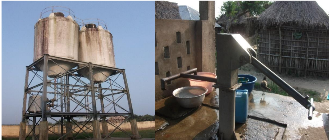
Plate 1: AEV installed in the town of Aguégués
