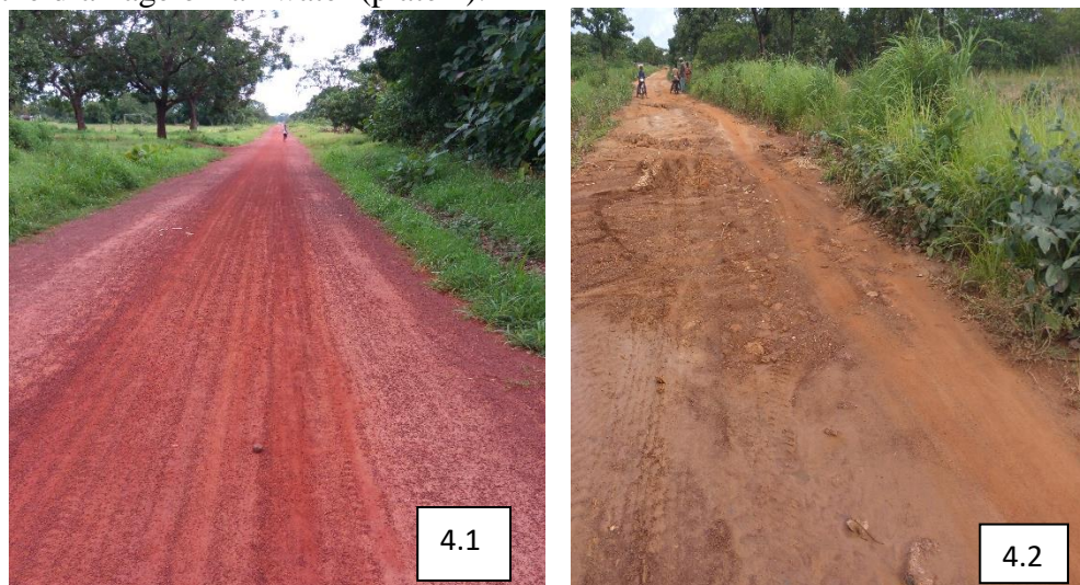
Plate 4: Road maintenance in the Commune Shooting: Anagonou, May 2021
