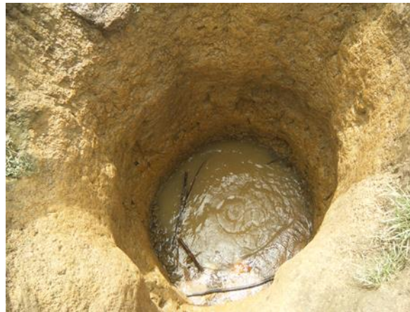
Photo 5: Partial view of the wall of a traditional well in Kerou
