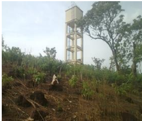
Photo 3: Water tower in Firou
