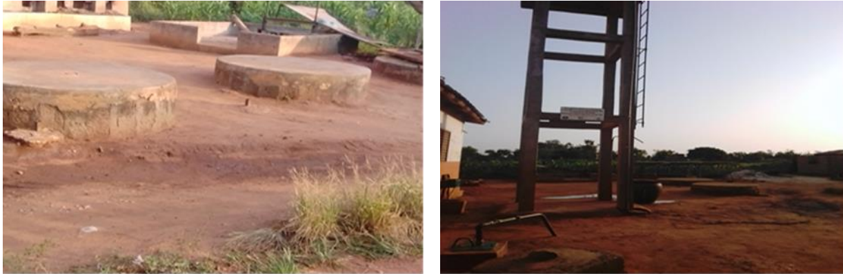
Plate 3: Partial view of waste management devices and infrastructure
